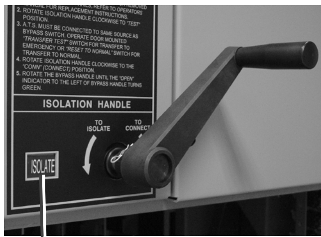
Figure 3-12. Isolation Handle turned to ISOLATE .
