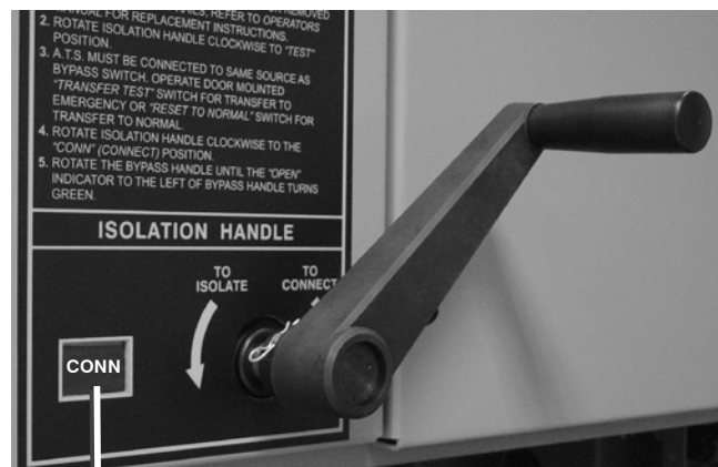
Figure 3-21. Isolation Handle turned to CONN .
