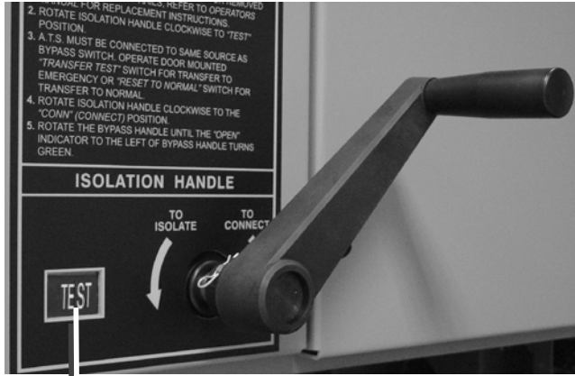
Figure 3-19. Isolation Handle turned to TEST .
