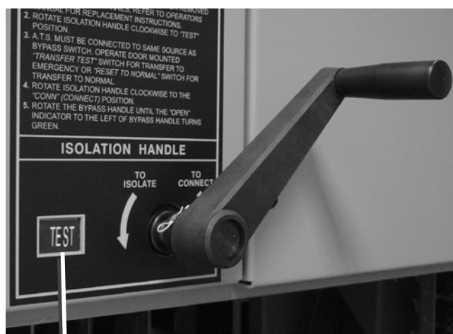
Figure 3-10. Isolation Handle turned to TEST .
