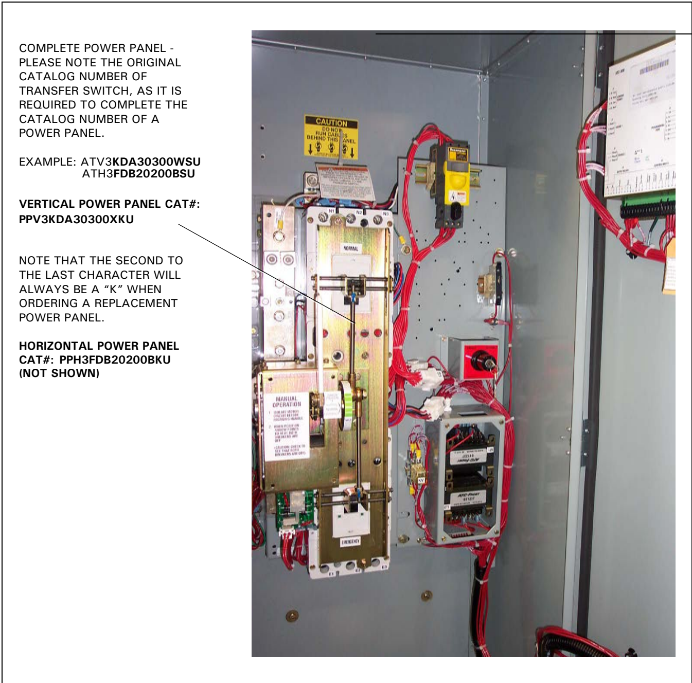
Figure 36A Typical ATC-300 Controlled Breaker Based ATS.
