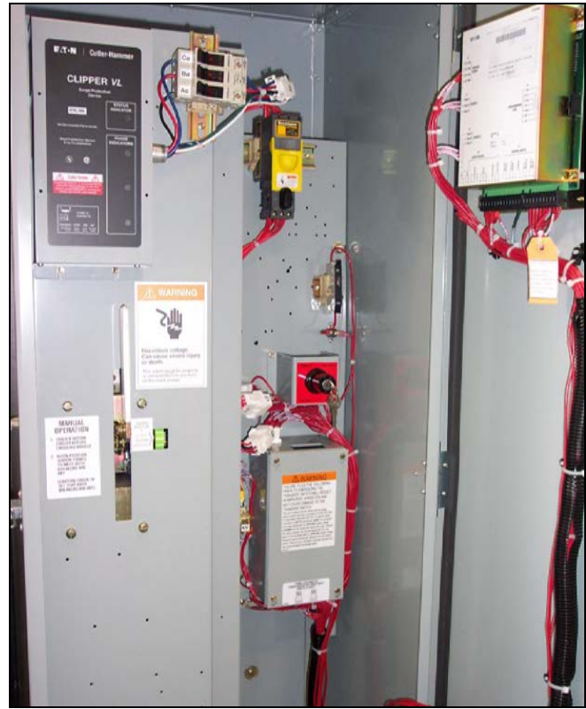
Figure 5. Vertical Design Transfer Switch with the Deadfront Cover in Place Over the Power Panel (225-1200 A).
