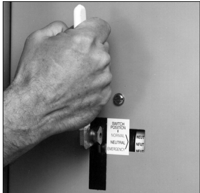
Figure 31. ATS Manual Operating Handle in Use (225-1200 A Models).
